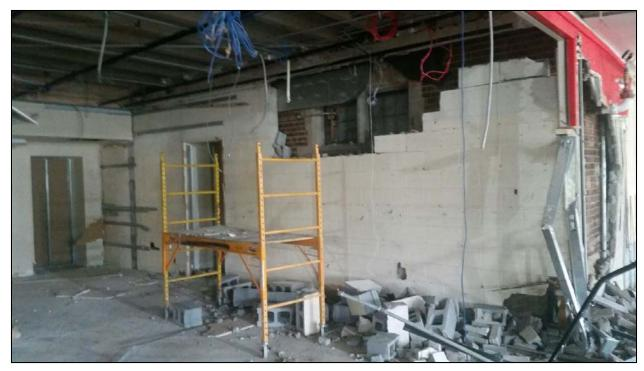
The original 1927 building was covered with concrete blocks when the 1960s addition was added. The blocks have been removed and this wall of the original Library will be restored and exposed. One window in the center of the wall was removed in 1980. This portion of the wall will be replaced with brick. This particular area of the wall is the future home of the Circulation staff office.
