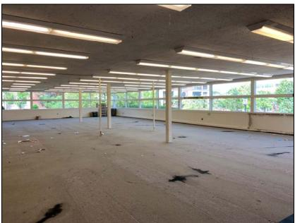
The Dailey Company began construction with the removal of the fire suppression system from the ceiling and demolition of walls, ceiling tiles, and carpeting.
