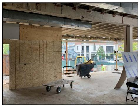
Welders have been working to remove the exterior wall of the Youth room. After 4 days of work, the windows and mullions have been removed on the north wall.
