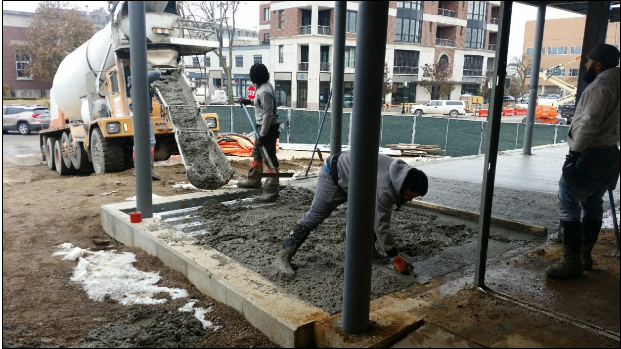
The concrete floor in the addition area was poured on November 20.
