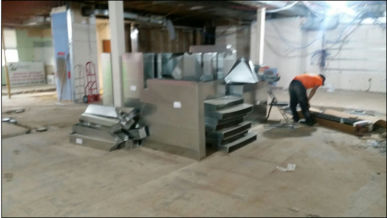
The sheet metal for ductwork was delivered and is being formed into vents and hung throughout the space.
