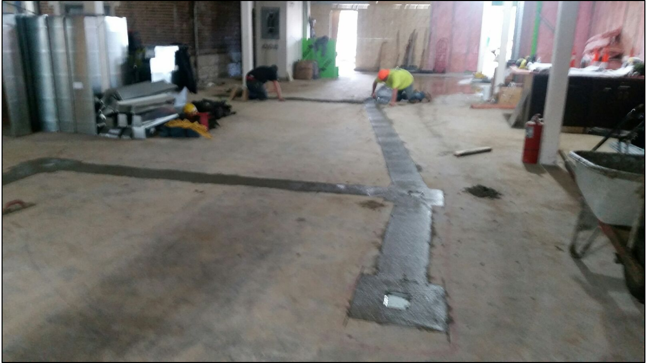
The trenches were filled in with concrete on December 4.
