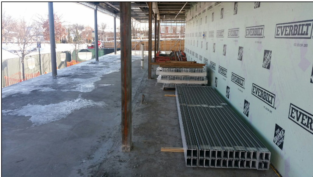
Steel for curtain wall
