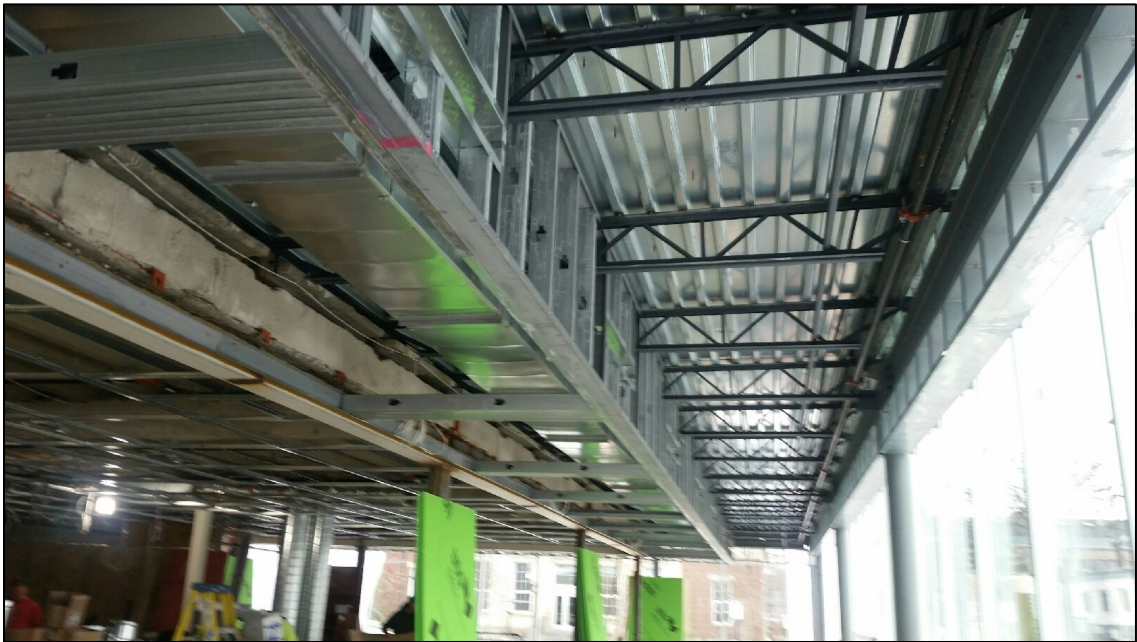
View of ceiling detail along the curtain wall. The outer perimeter of the Youth Room will have higher ceilings than the main portion.
