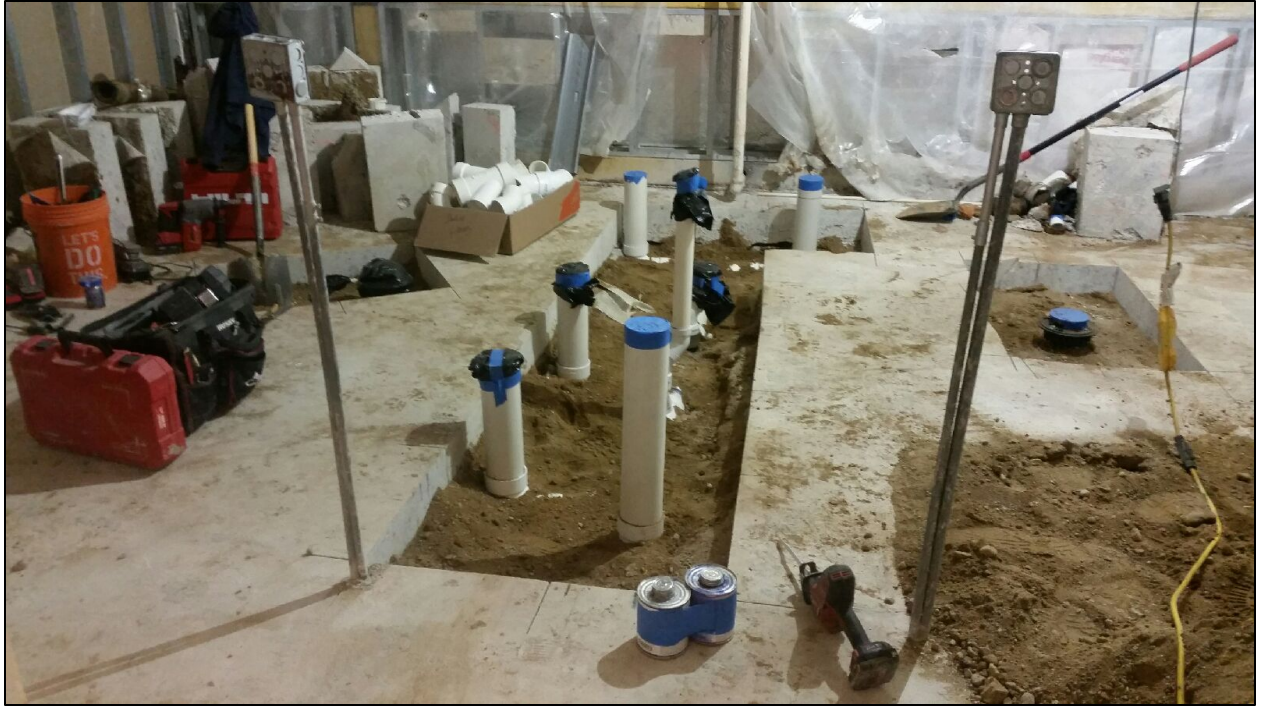
Plumbing installation in restrooms
