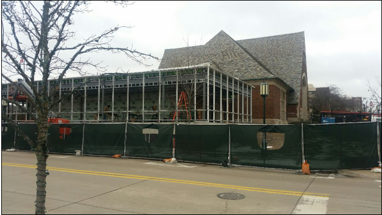
Curtain wall frames in place just prior to window installation.
