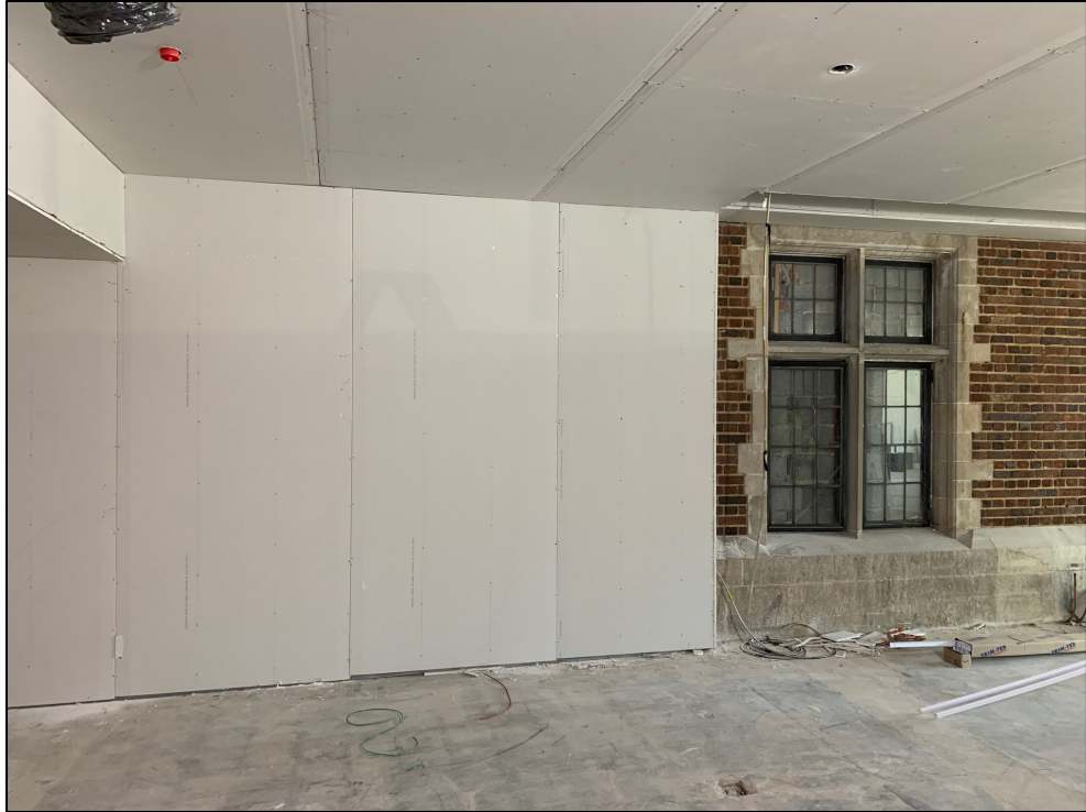
Looking north toward the Circulation staff office wall. The window has been preserved and the new split HVAC system is housed behind the drywall.
