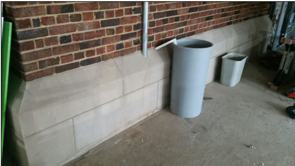
Newly repaired limestone base on the original 1927 exterior wall.
