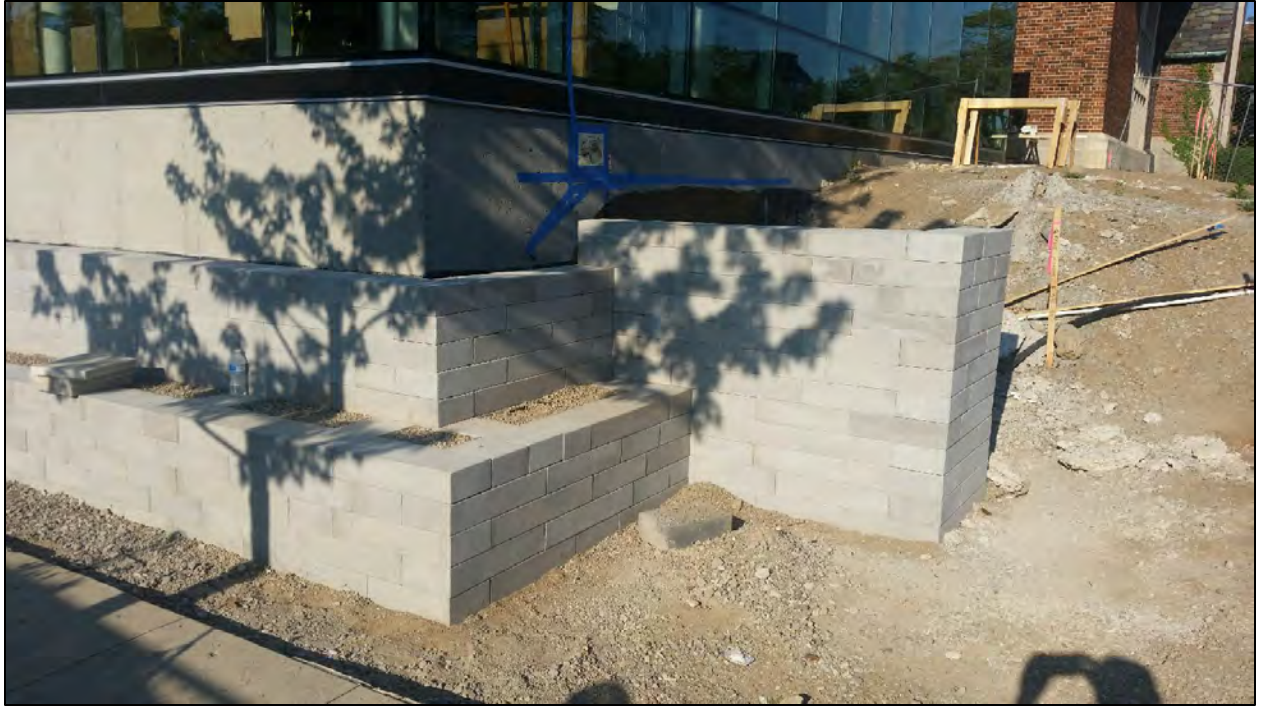
Work on the retaining wall continued and fill dirt was added to grade the Children's garden.
