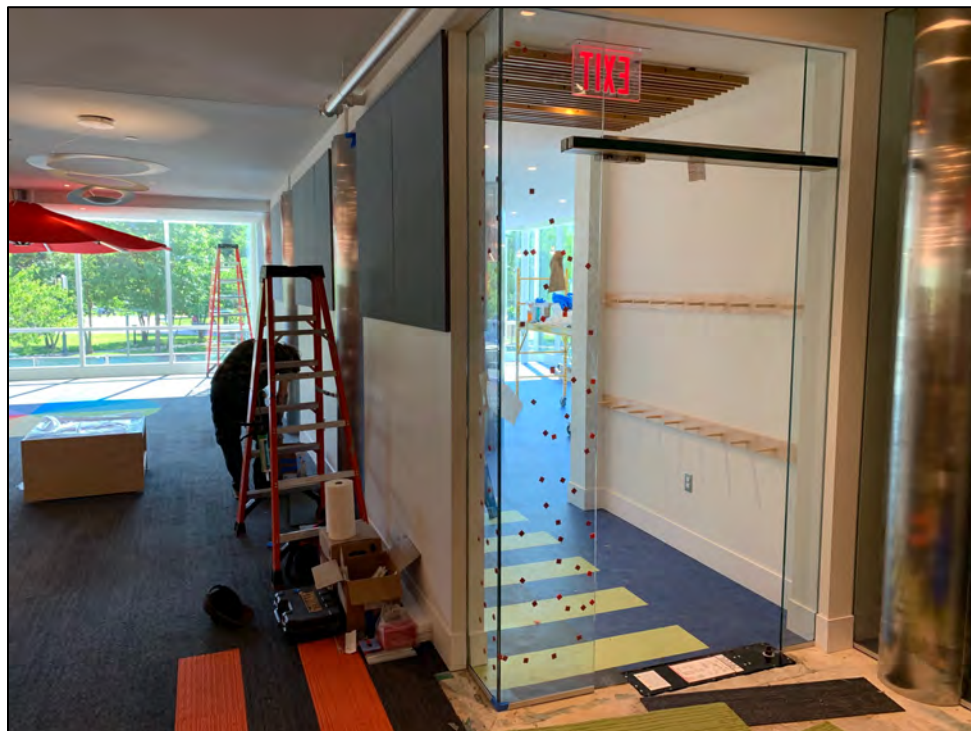
Glass doors and walls were added to the space on July 16 and 17. The door to the Discovery Room will have an electronic door with an automatic door opener.
