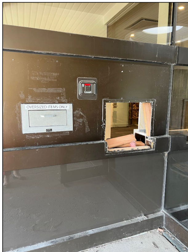
View of exterior book drop after removal of door.
