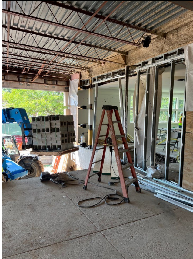
Masonry bricks loading into the building for elevator pit walls.
