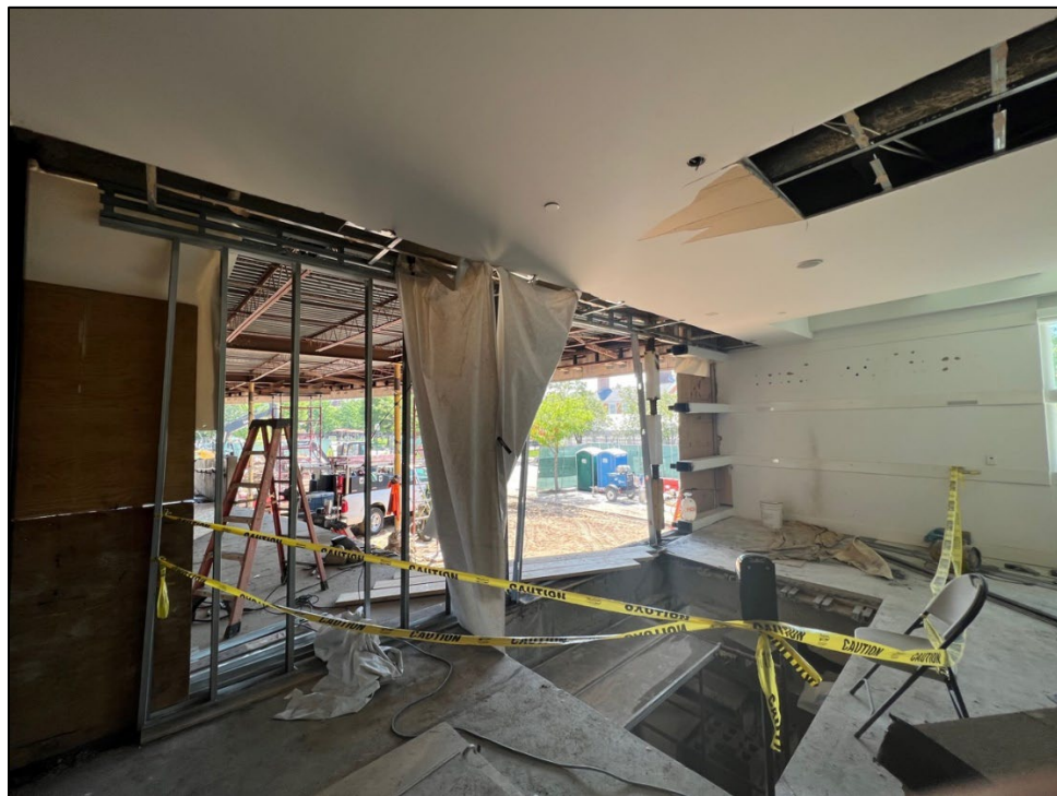
Former exterior walls removed. Elevator pit excavation.
