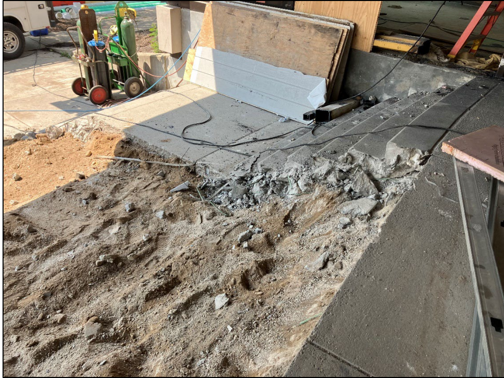
Removal of the entry steps in progress.
