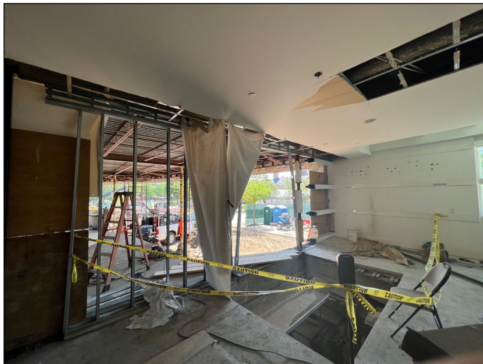
Former exterior walls removed. Elevator pit excavation.
