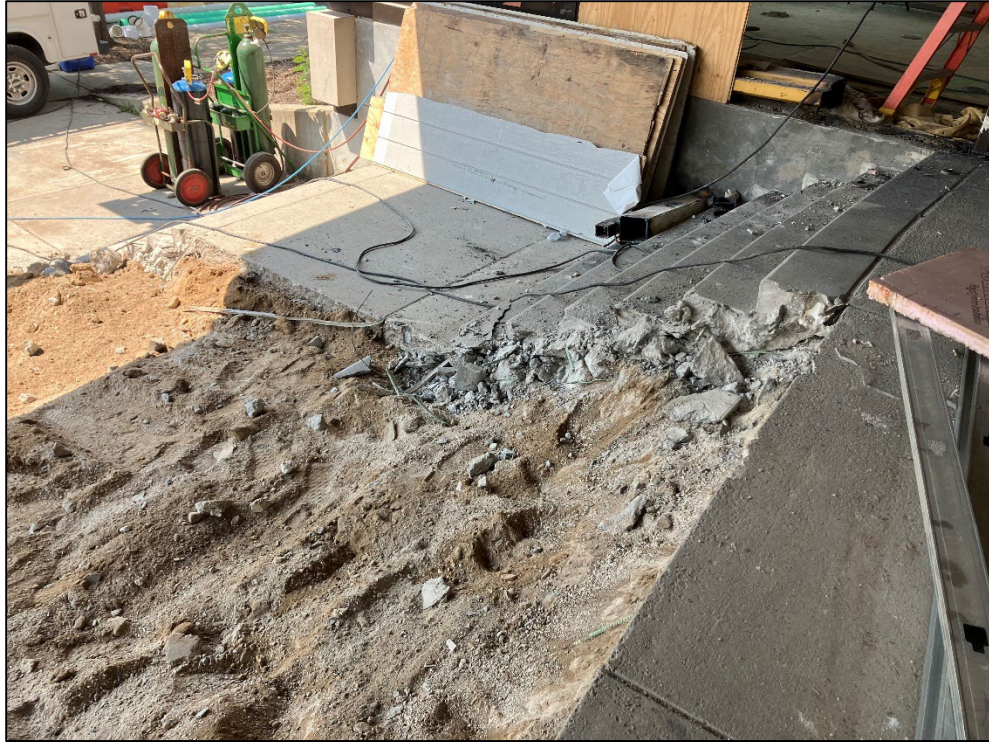
Removal of the entry steps in progress.
