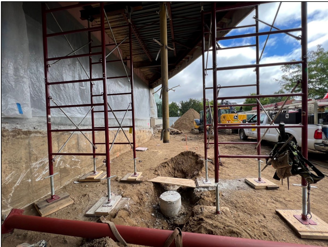
Looking at former support column shored up, cut, and ready for replacement.
