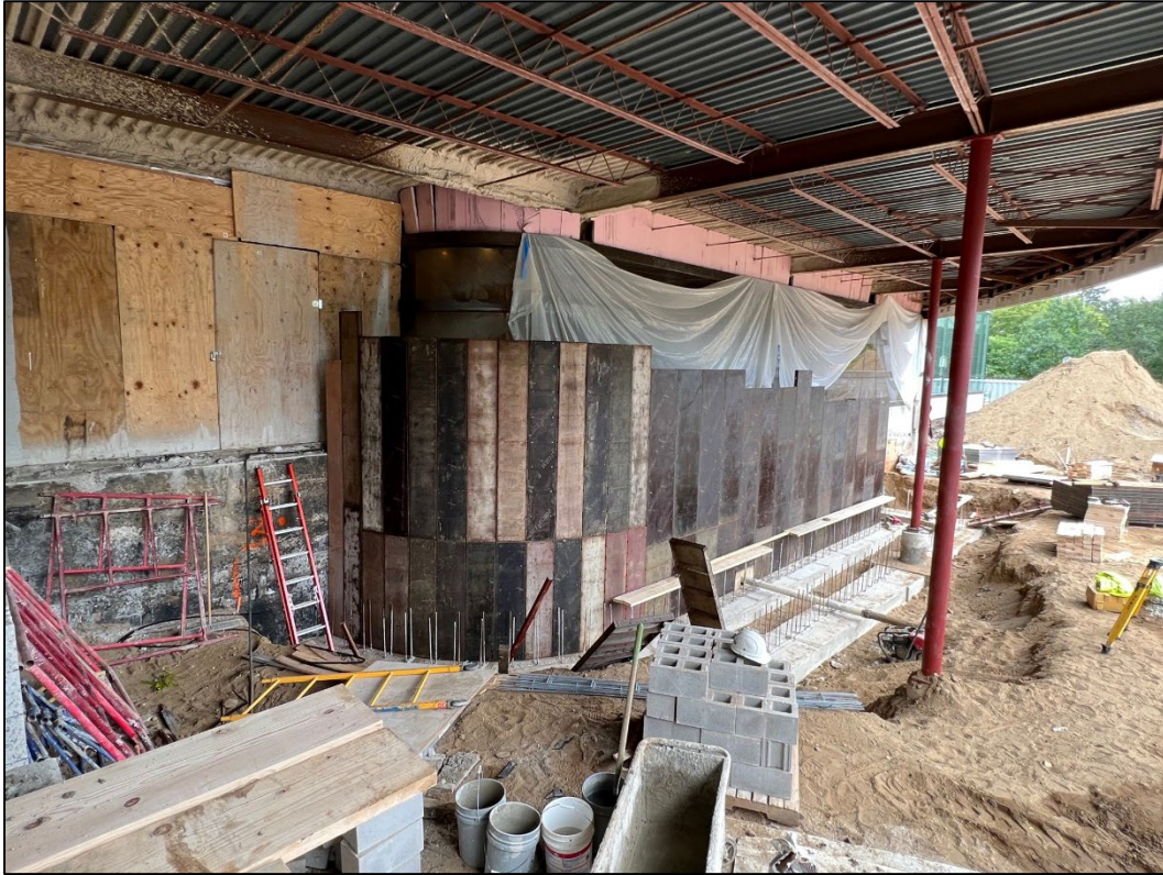
View of ramp concrete work. The tall curved wall is the middle wall of the new ramp.
