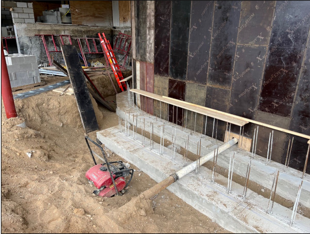
View of ramp footings near entrance to base of ramp.
