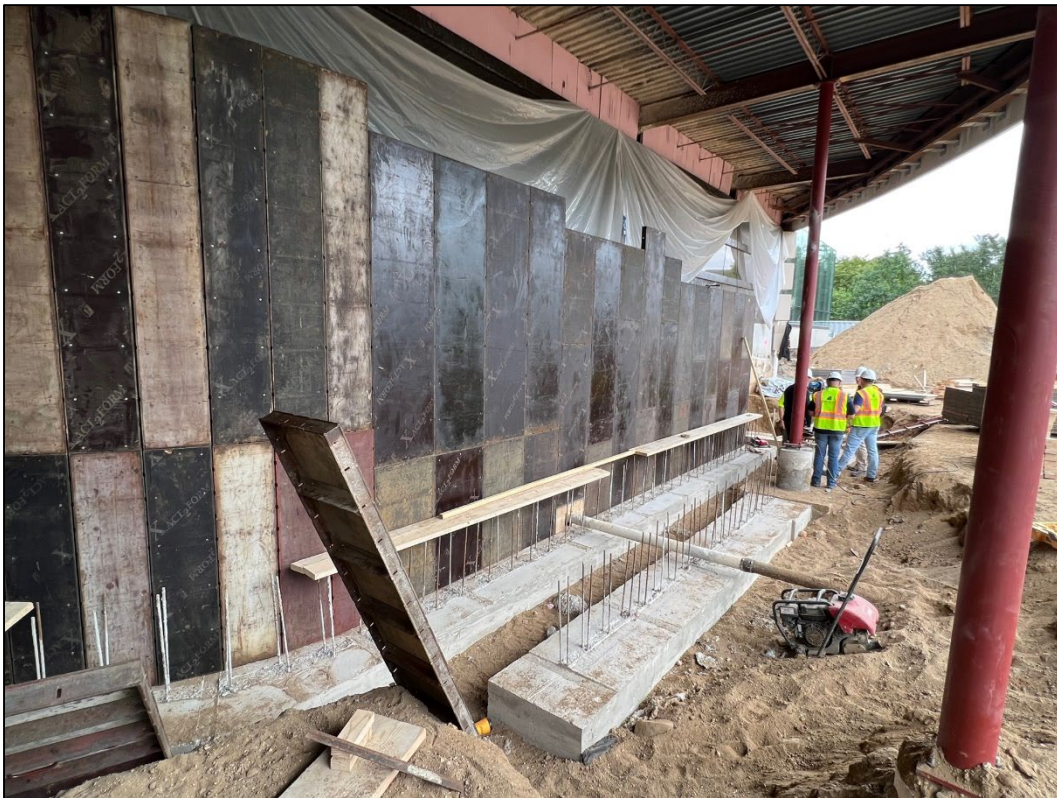
View of underground ramp footings and rebar set in place for new ramp base and walls.
