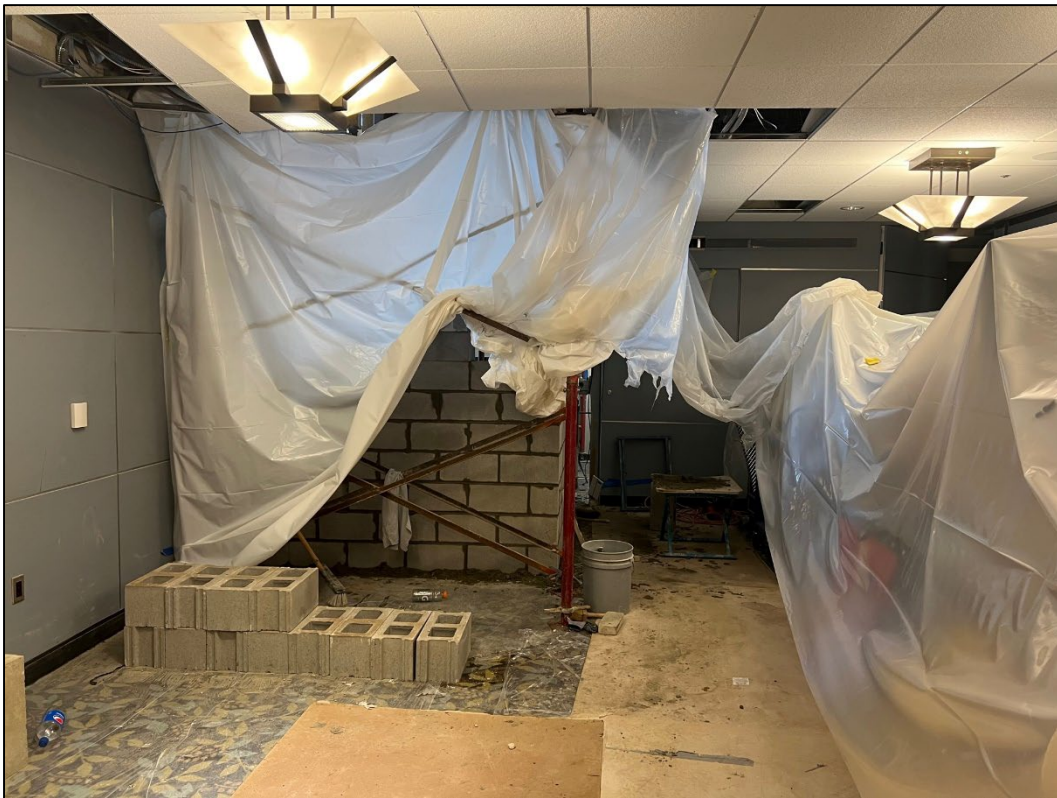
View of new elevator shaft being built in the corner of the Rotary Room
