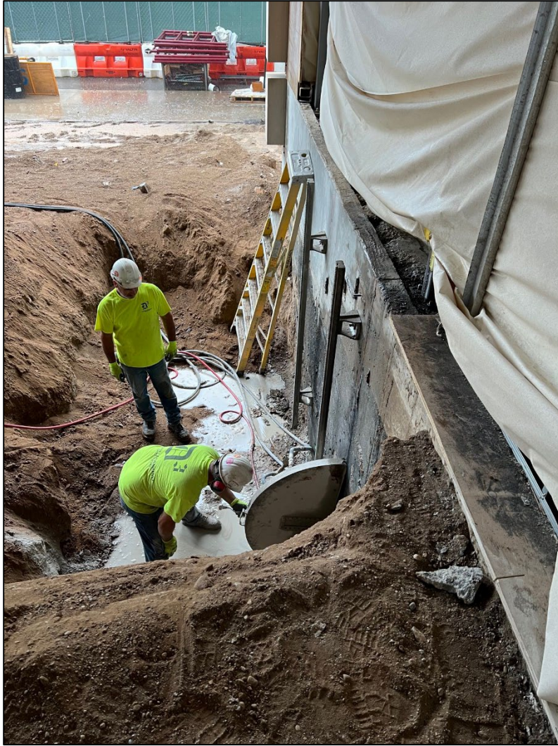
Workers saw cutting the foundation for the new elevator door on the entry level.
