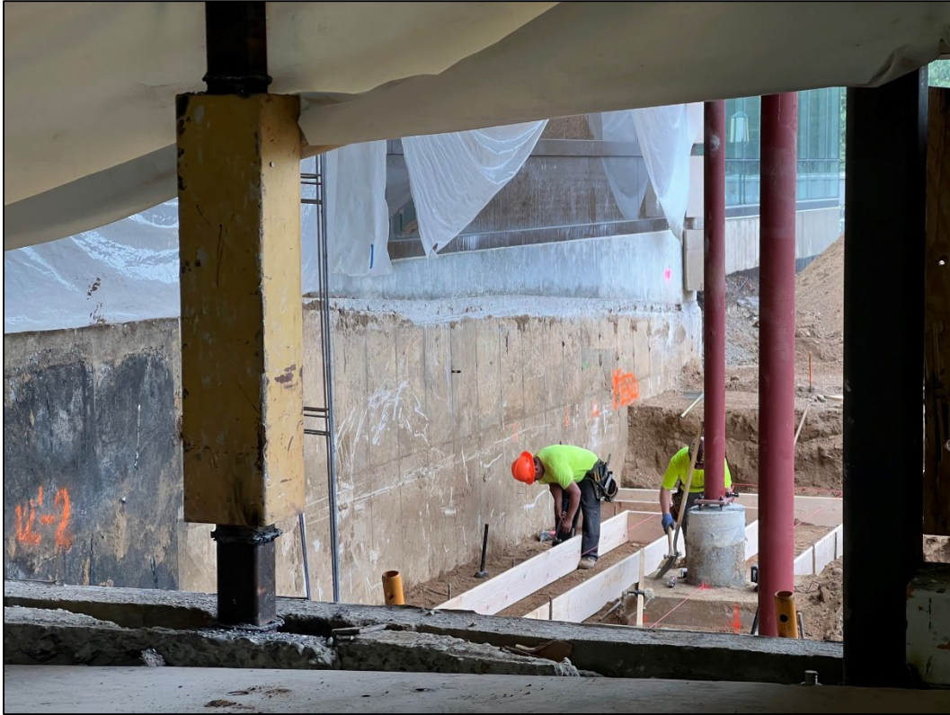
View of footings being poured for new interior ramp.
