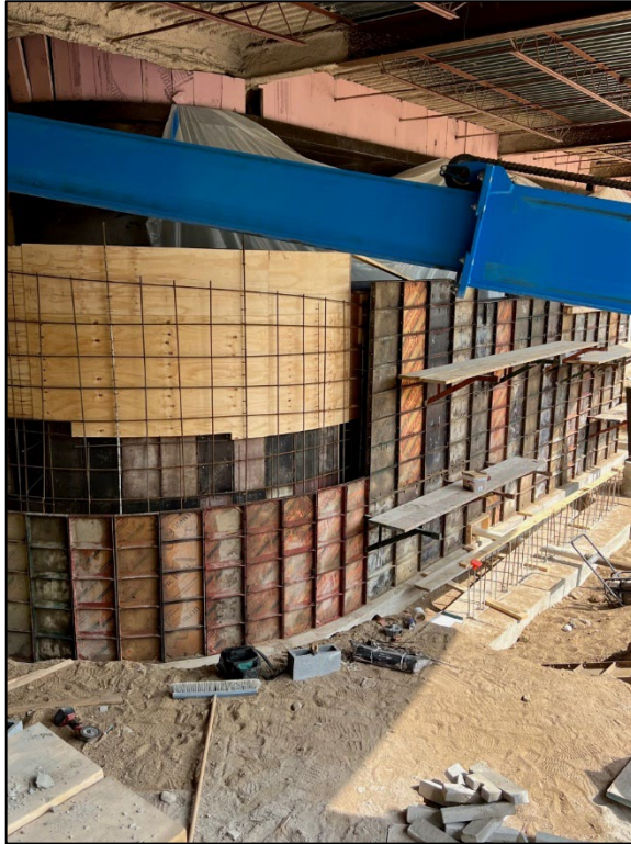
Concrete forms for new ramp in progress.
