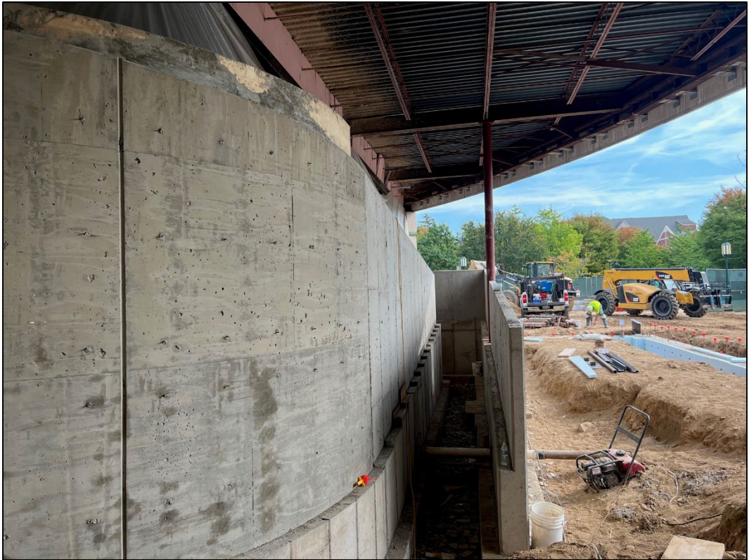
View of new ramp walls in progress.
