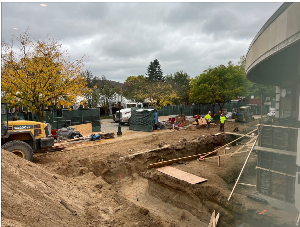
View of excavation in progress for new footings.
