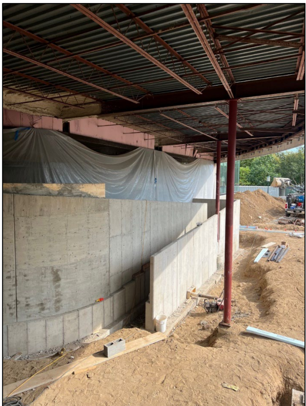
View of new ramp walls in progress.
