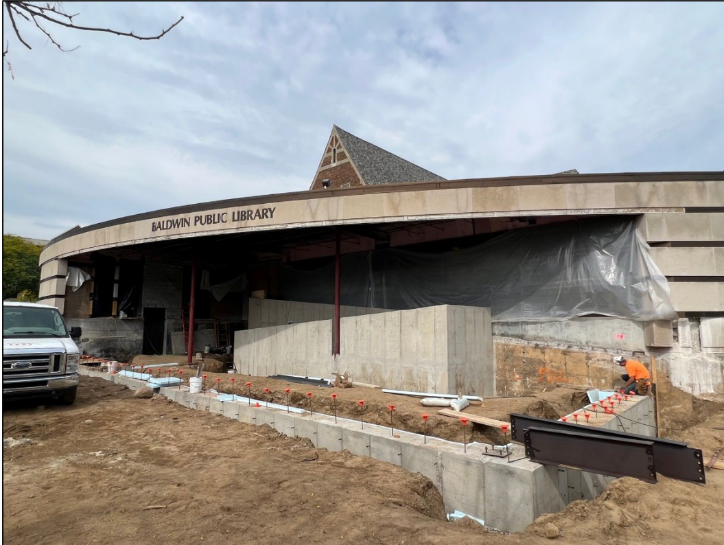
October 4, 2023: View of footings for exterior addition and concrete ramp walls.
