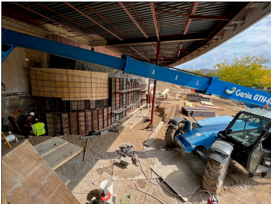
Concrete forms for new ramp in progress.
