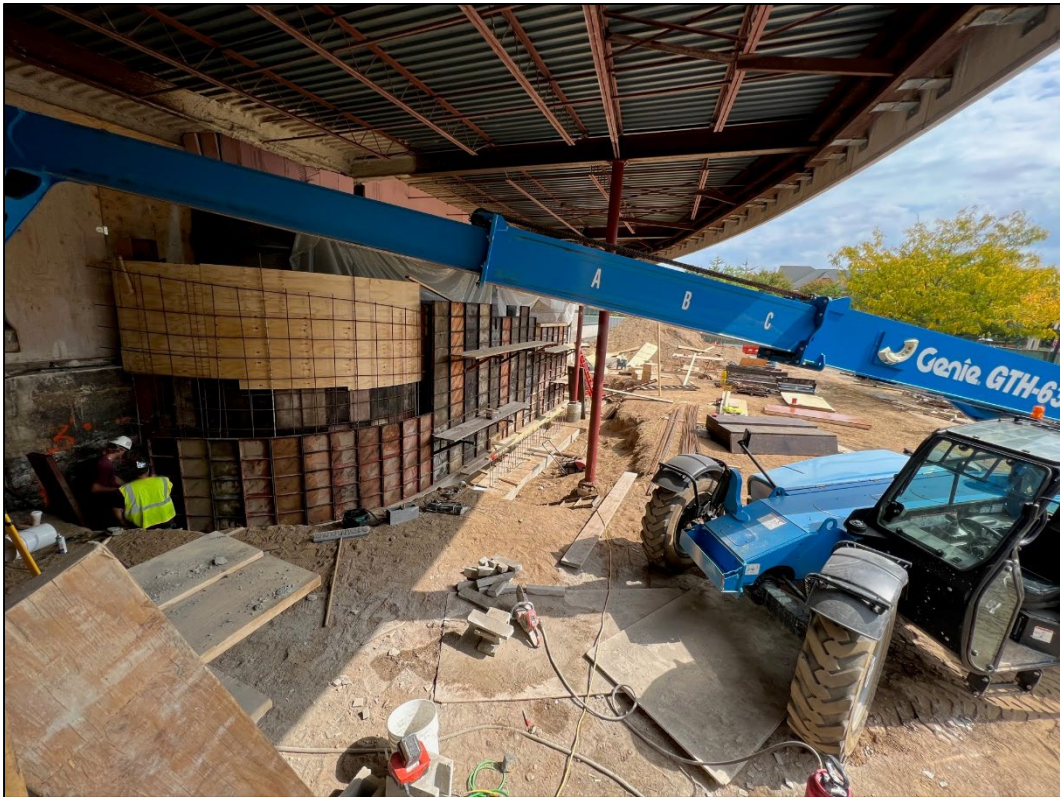
Concrete forms for new ramp in progress.
