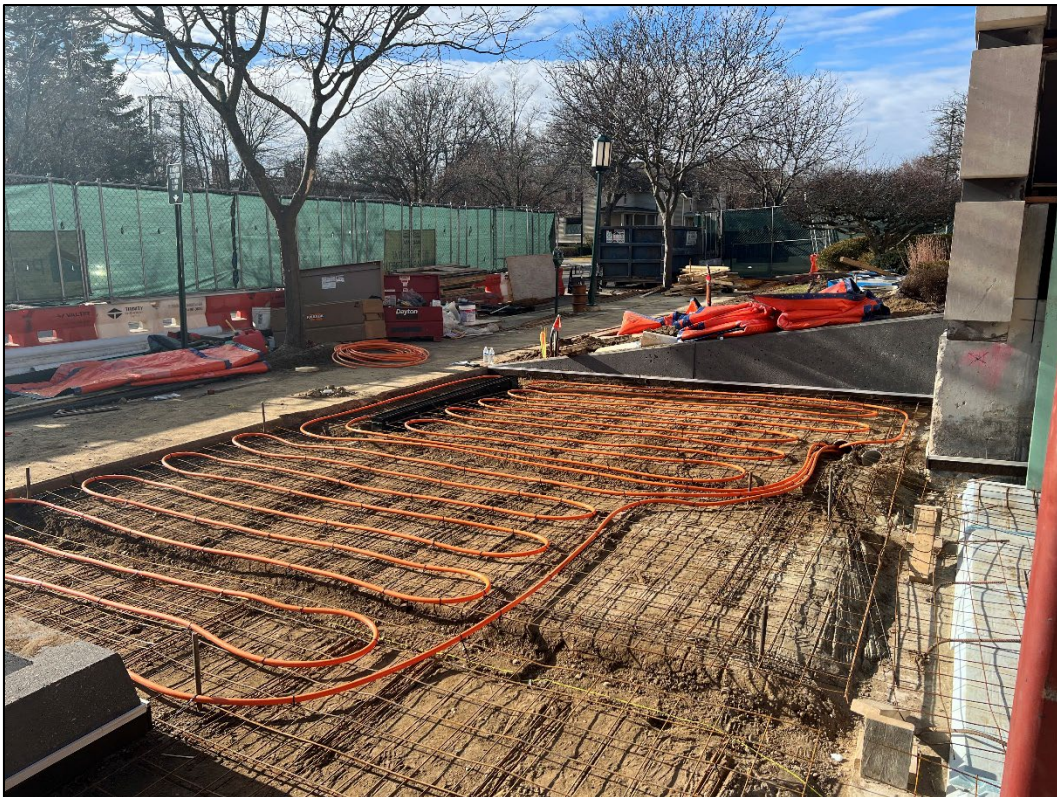
View of snowmelt system installation progress
