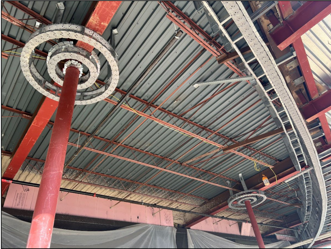
View of ceiling framing around original columns of Birkerts awning
