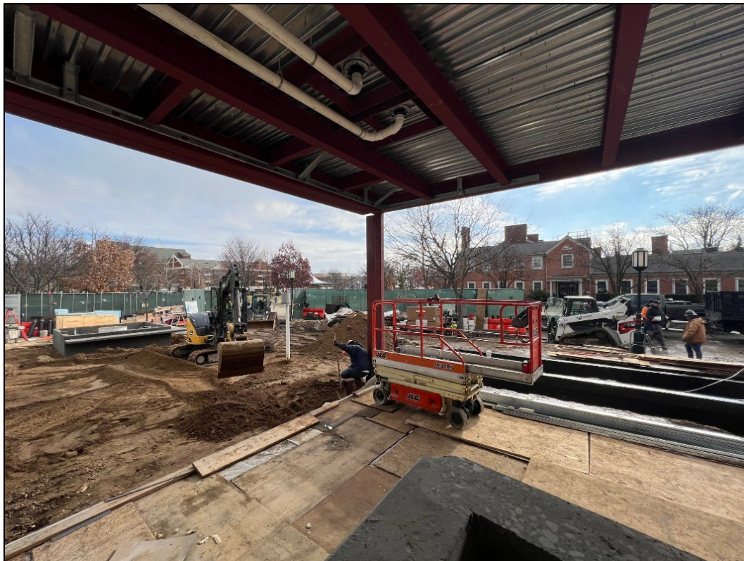
December 6, 2023: Southeast corner of the addition. Note the drains from the roof to new underground detention system
