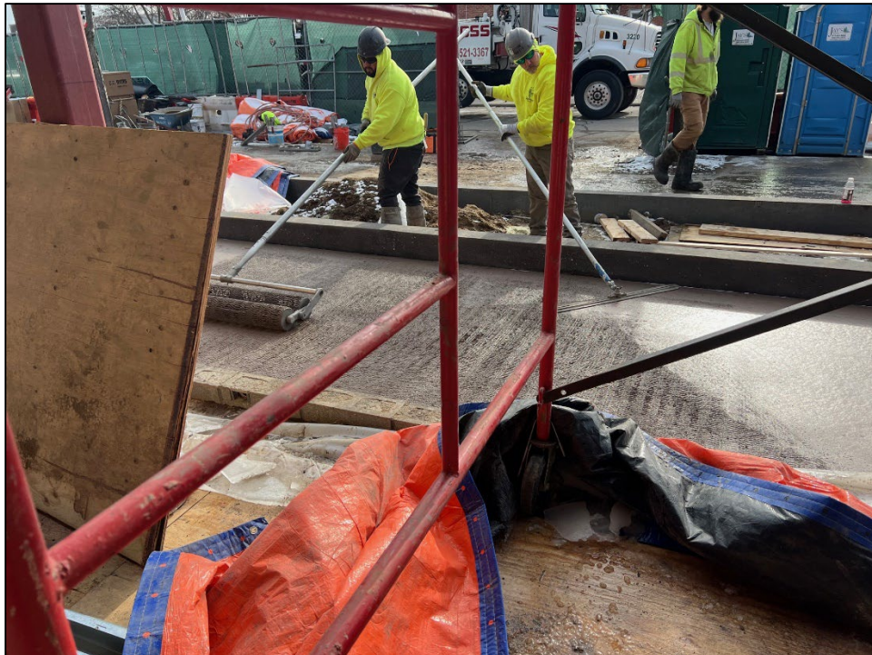
Concrete installers push larger aggregate lower in order to have a more uniform surface
