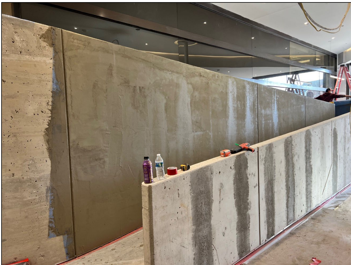
Ramp wall plaster in progress
