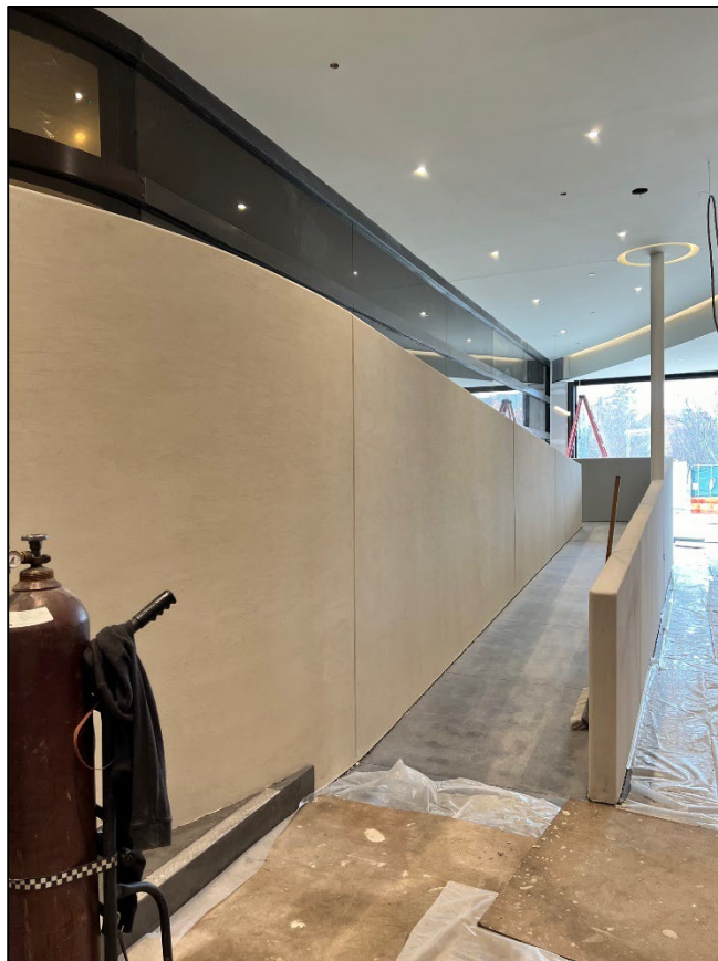
View of plaster on ramp
