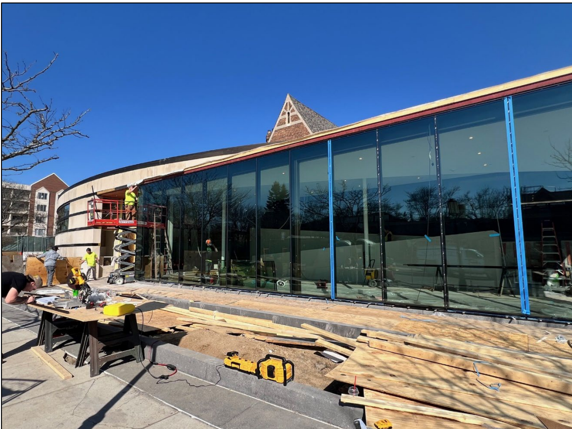
Window caulking in progress
