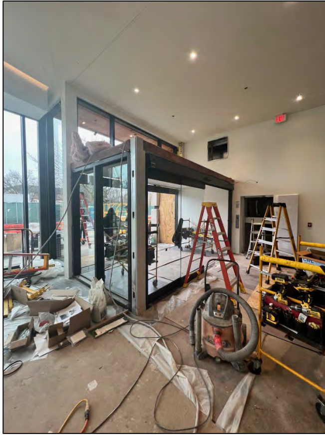
Automatic sliding doors installation in new vestibule
