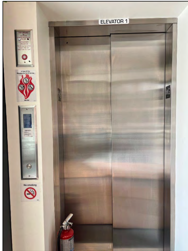
View of entry elevator doorway
