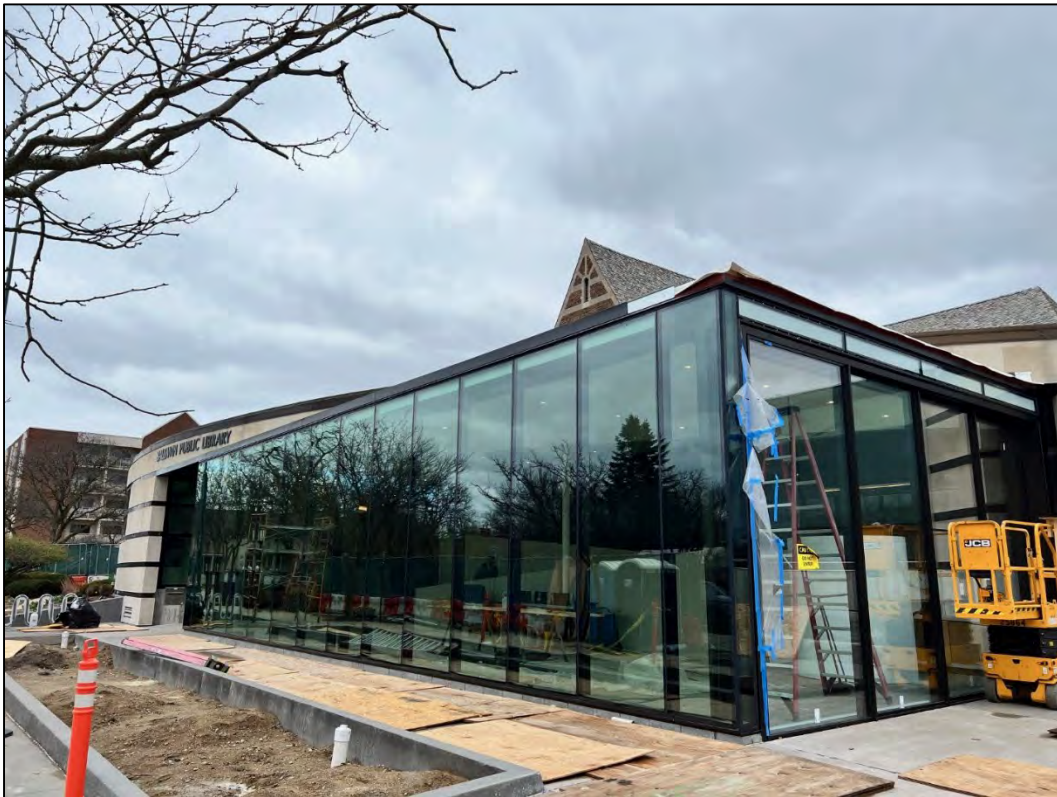
View of addition exterior from corner of Merrill and Bates
