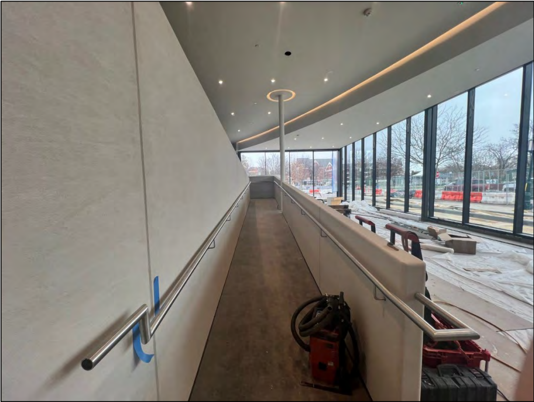
Handrail installation on new ramp
