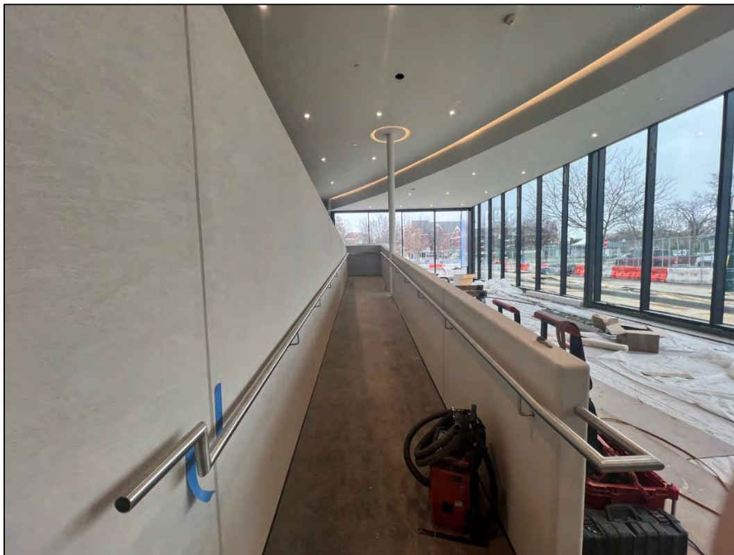
Handrail installation on new ramp
