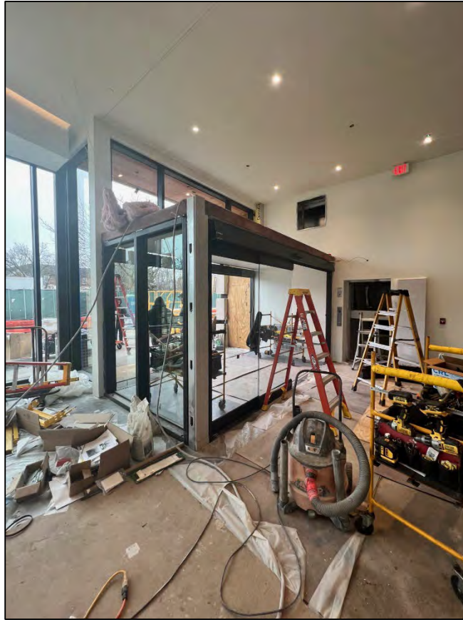
Automatic sliding doors installation in new vestibule
