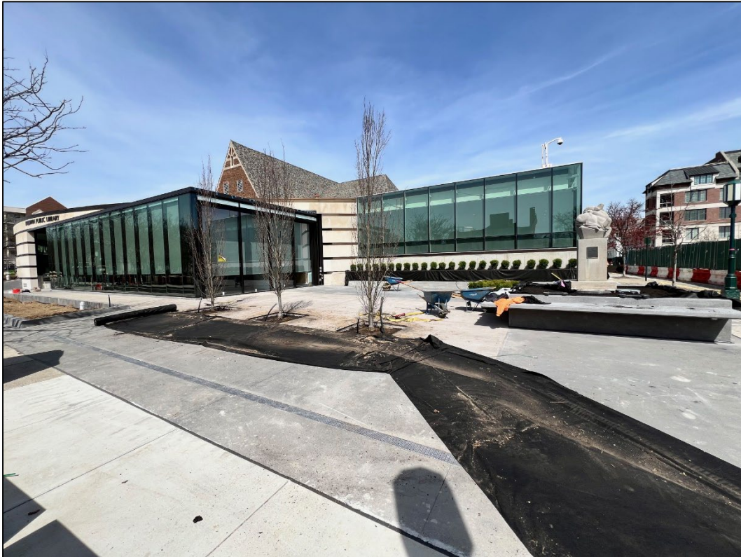
New outdoor plaza landscaping in progress
