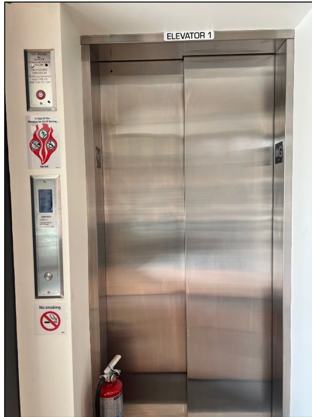
View of entry elevator doorway
