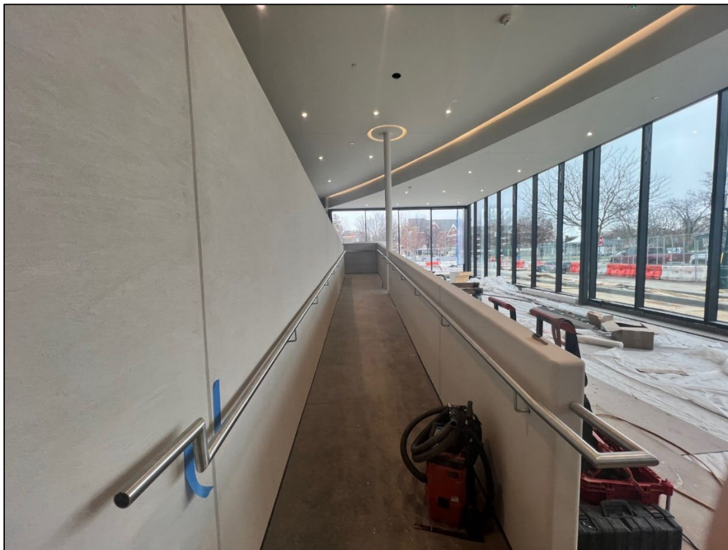
Handrail installation on new ramp
