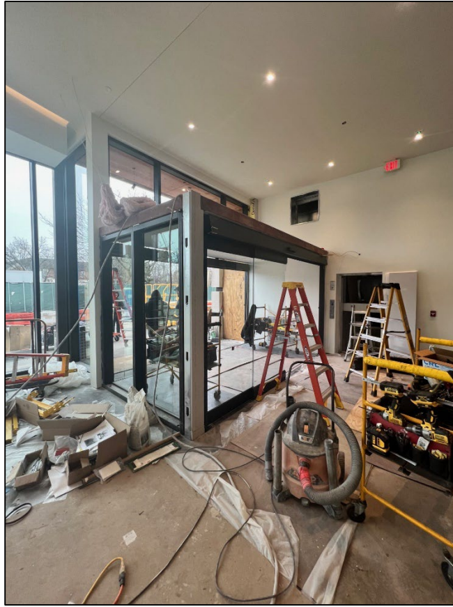
Automatic sliding doors installation in new vestibule
